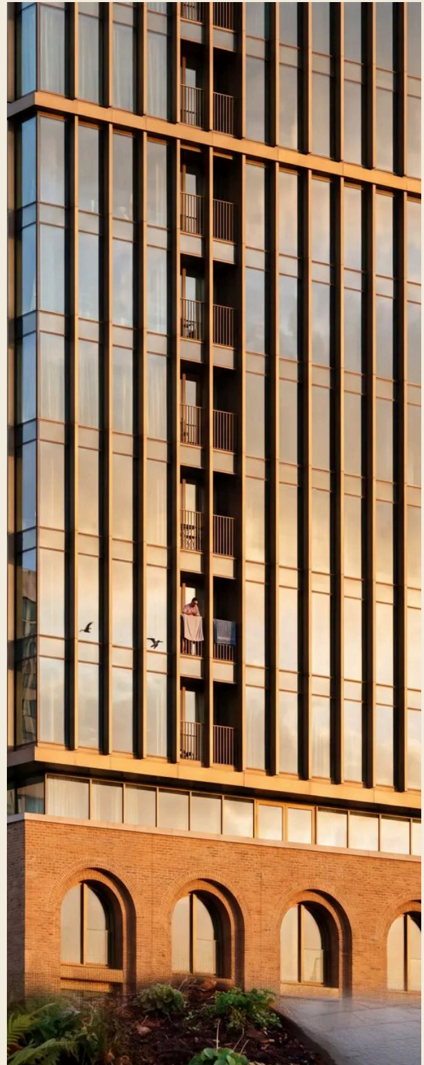
TEN FLOORS OF THE SHAFT AT REAL SCALE — THE FINS, AND THE TOP OF THE BRICK BASE BELOW.
